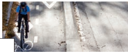
Bike lane separated by a raised curb; physical separation from through traffic or parking; cyclists can enter/exit at fewer locations and cars are blocked from entering
