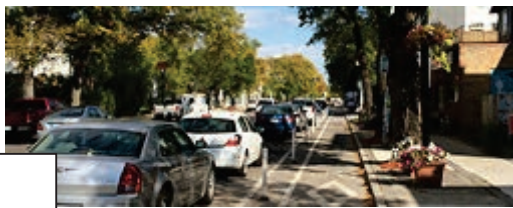
Bike lane separated by parking; horizontal separation from through traffic; cyclists can enter/exit at fewer locations but are vulnerable to illegal car parking
